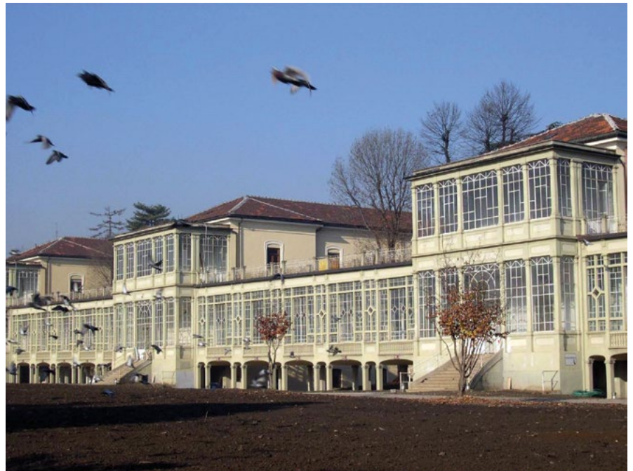
Fig. 12 – Former Riberi Hospital in Turin, the glass gallery and the central garden, after the restoration (2006)
