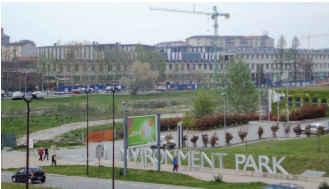
Figura 1. Vista di Envi Park. Figure 1. View of the Envi Park.
